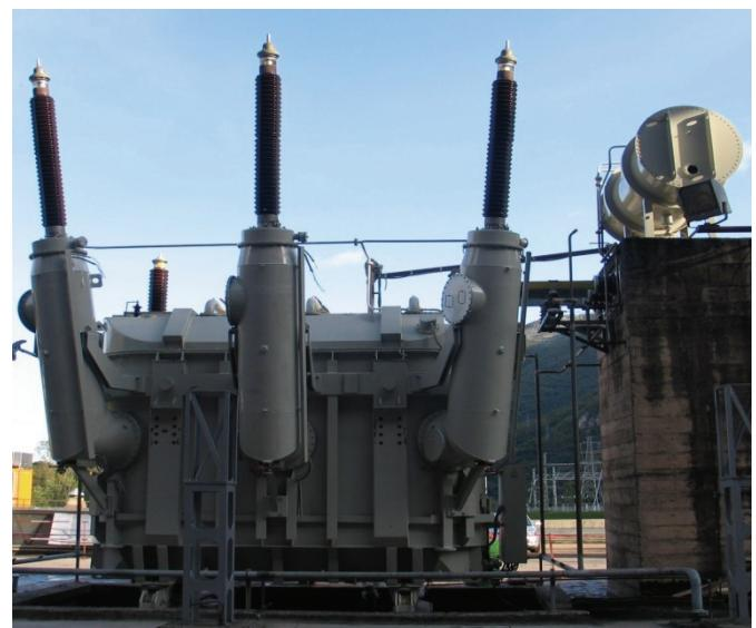
Fig. 1 Step up transformer 112 MVA
